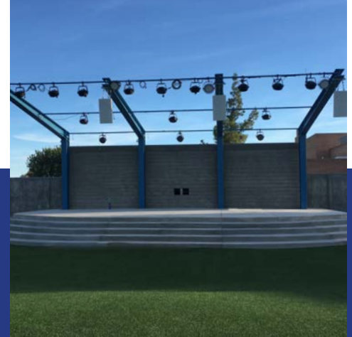
PALOMA OUTDOOR AMPHITHEATER TEMPE, AZ Audio & Lighting Installation
