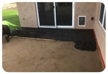
FlexTrail<sup>™</sup> can be installed right over top of most existing surfaces with little or no excavation required.
