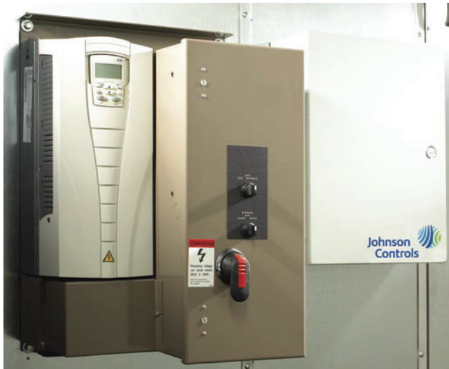
Variable-speed drives offer dramatic fan-energy savings.
