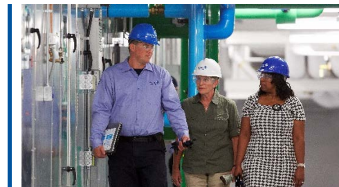
These activities are performed in order to gain as complete an understanding of the building operation as possible because, without this in-depth knowledge, improvement and savings projections could be meaningless.
