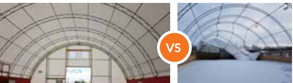
Britespan's 11 runs of 2 7/8" 14 ga purlins. Double 5/8" bolt connections
