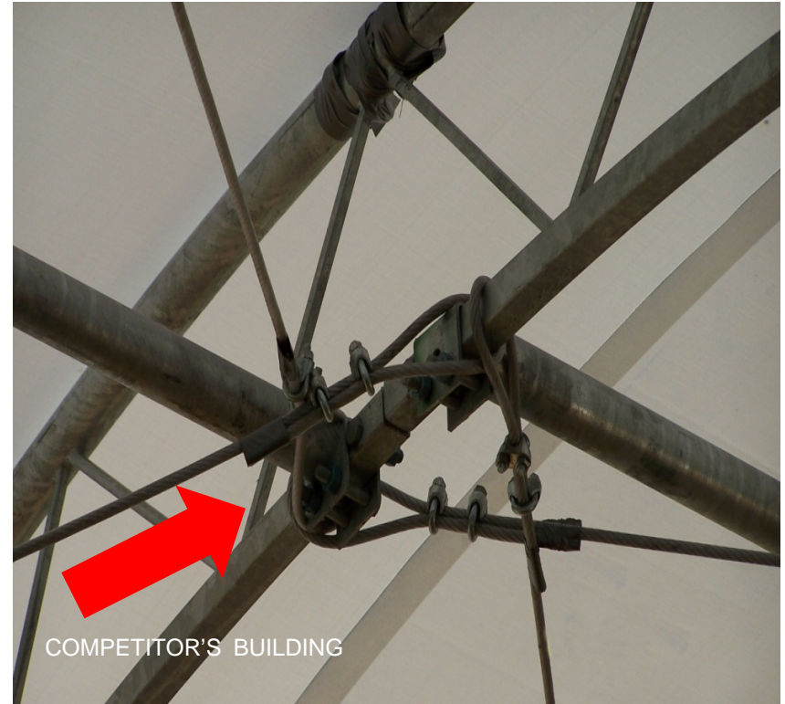
CABLES WRAPPED AROUND SADDLE BRACKETED PURLINS
