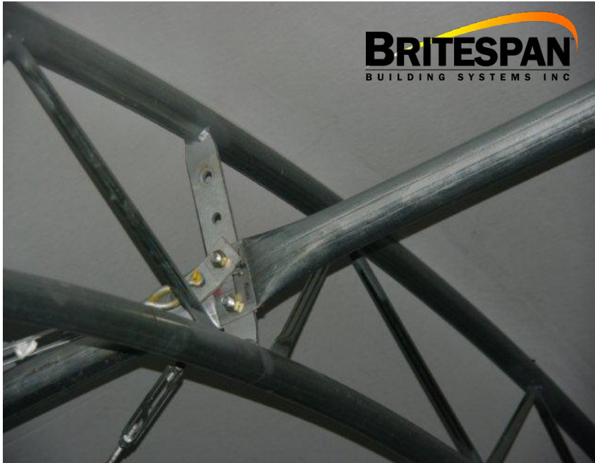
DOUBLE-BOLTED TO AN ENGINEERED STRUCTURAL MEMBER
