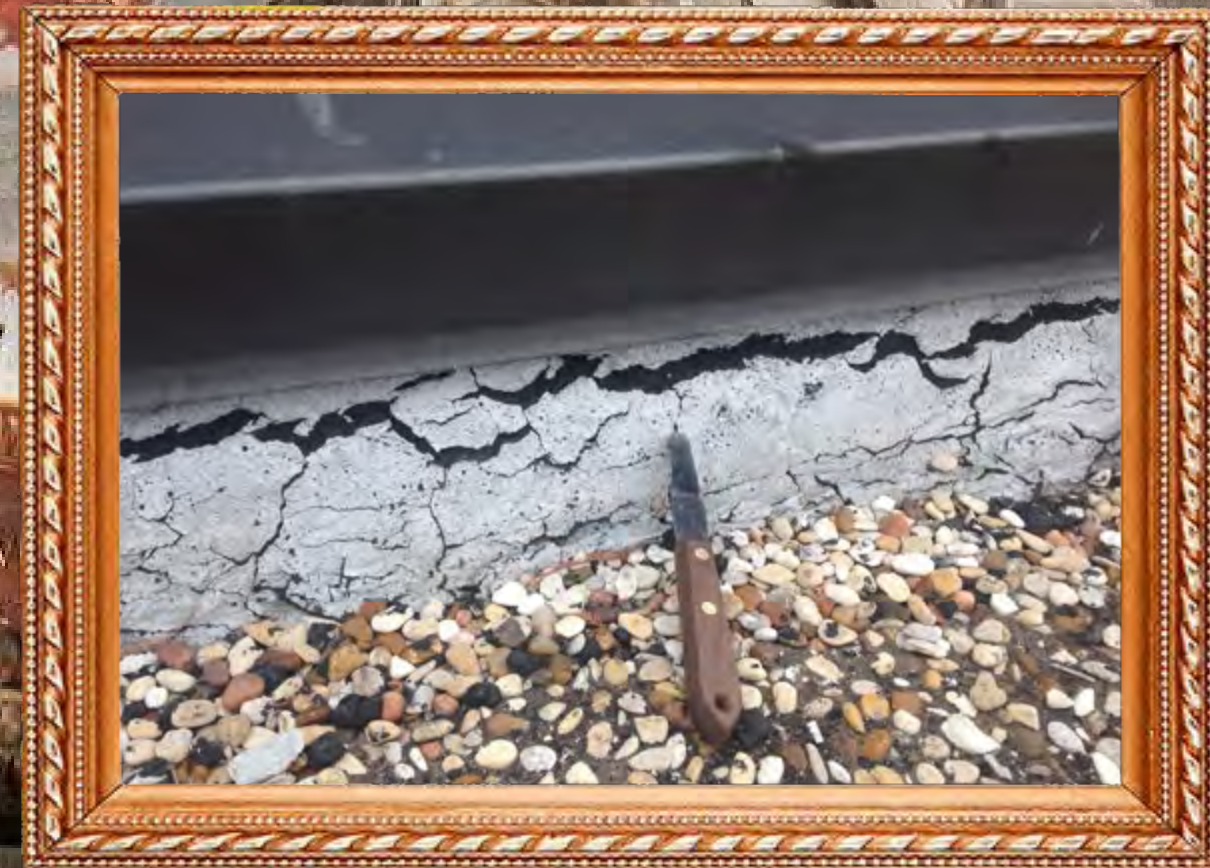
Existing coal tar pitch roof was improperly repaired causing pre-mature roof system failure
