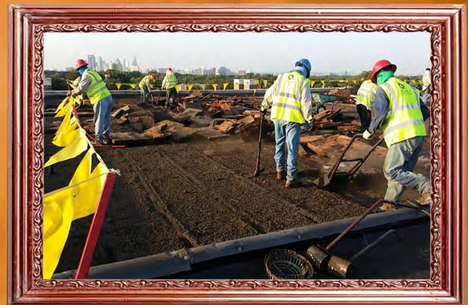
Removal of the phenolic insulation
