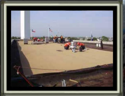
*Square Cut Into Existing Roof Kept Water Tight During Entire Project*
