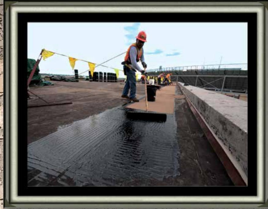
*Cold Process of Cap Sheet Instal*
