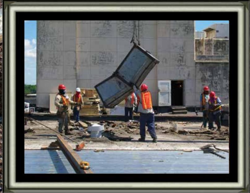
*Castro Roofing was commissioned to cut a square into the existing roof in the main hall to allow other contractors attic access to upgrade the electrical and mechanical systems.*
