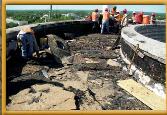
The original building was constructed in 1936 and many of the roof components were decades old. The flat roof drains were filled with debris that had accumulated through the years. Removing the old skylights revealed challenging conditions that required additional sheet metal work to assure a weather-proof seal. Working closely with the skylight subcontractors was essential.
