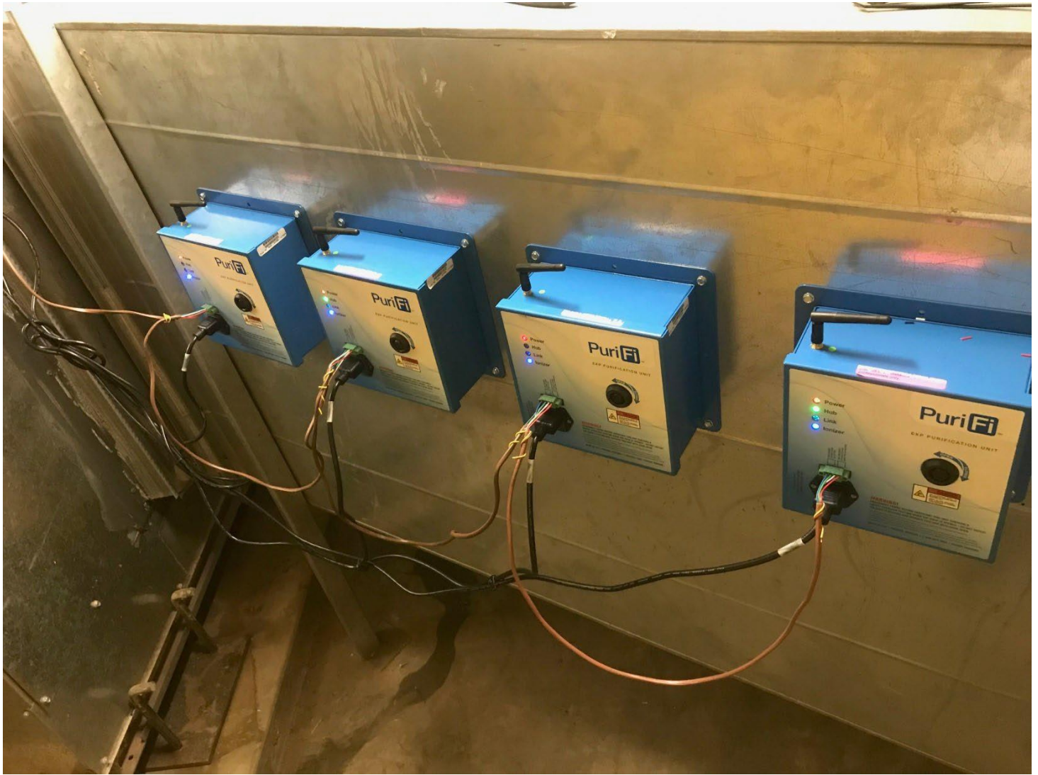
Multiple Marsden CleanAir units installed into a major duct work system in Tuba City Unified School District in northern Arizona.
