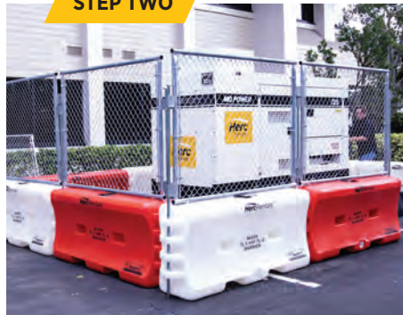
Fence and crash barrier
