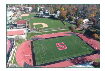
Swarthmore Colleges stadium was recently upgraded by The LandTek Group. The existing turf field was removed as well as improvements and reconstruction were done to the existing stone base. A new state-of-the-art synthetic turf field was installed along with updated athletic netting systems. The track was milled, repaved and striped with a fresh new look.
