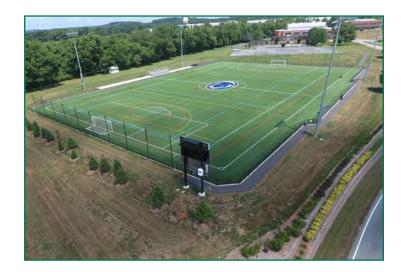
The new home of Penn State Harrisburg's mens and womans soccer team was constructed by The LandTek Group. The new construction of the multipurpose field included excavating the site and building a new drainage system and stone base. LandTek also installed perimeter fencing, a ball stop netting system, surrounding concrete walkways and a Musco lighting system.
