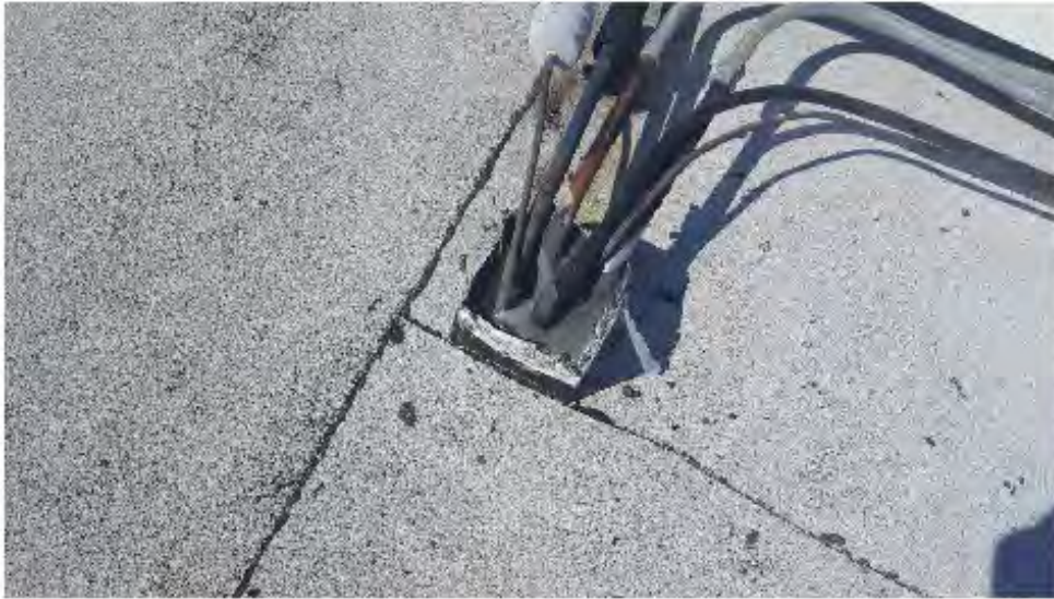
Low pourable sealer in pitch pan
