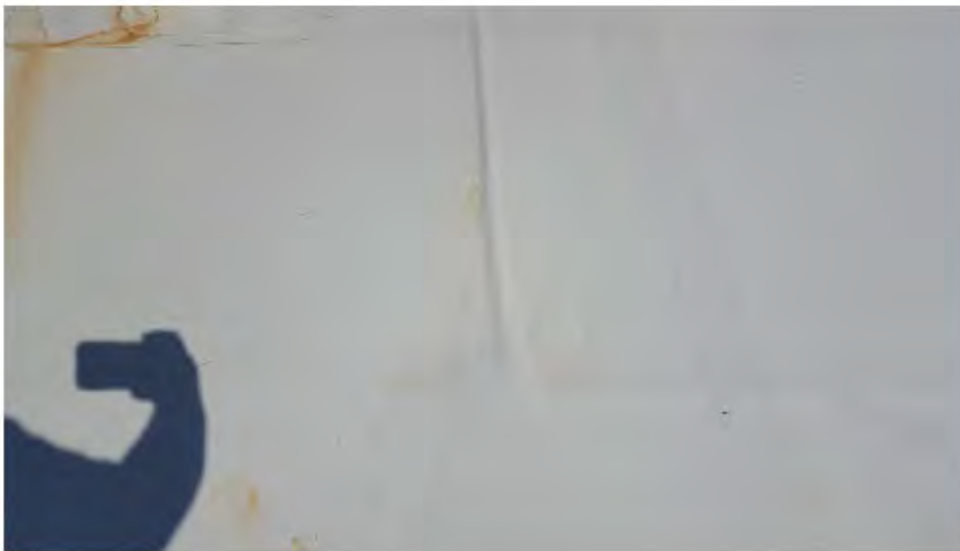
Ridging in membrane caused by loose insulation
