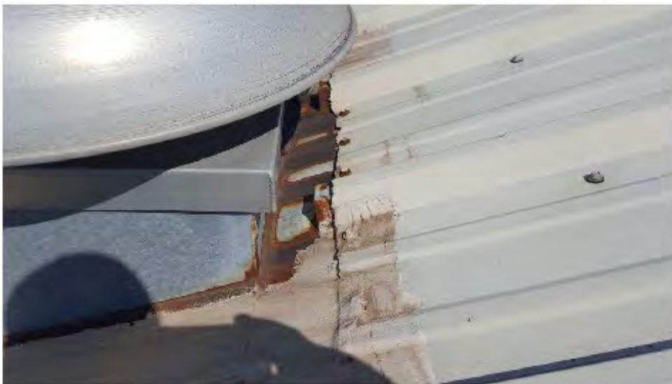
Rusted curb flange; rusted fasteners
