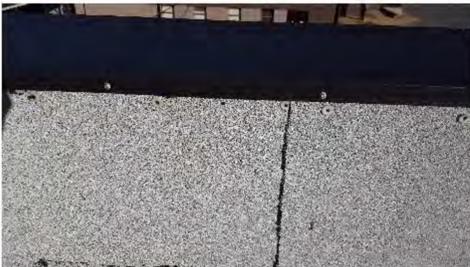
Exposed nails at wall flashing
