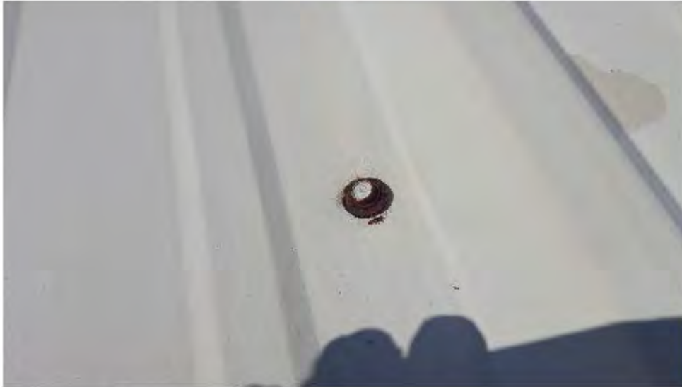
Rusted fasteners
