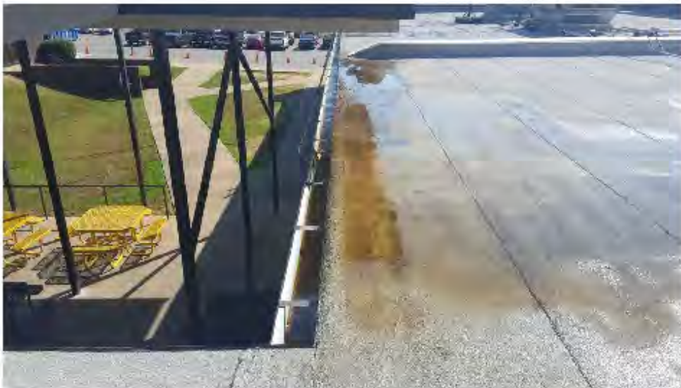
Ponding water resulting from leaking pipe
