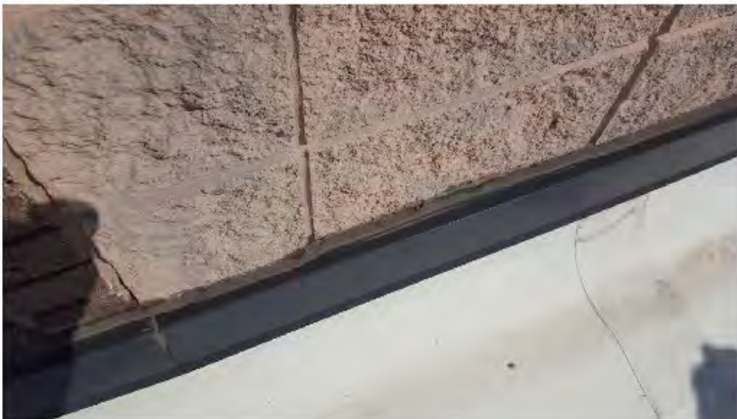
Deteriorating caulk
