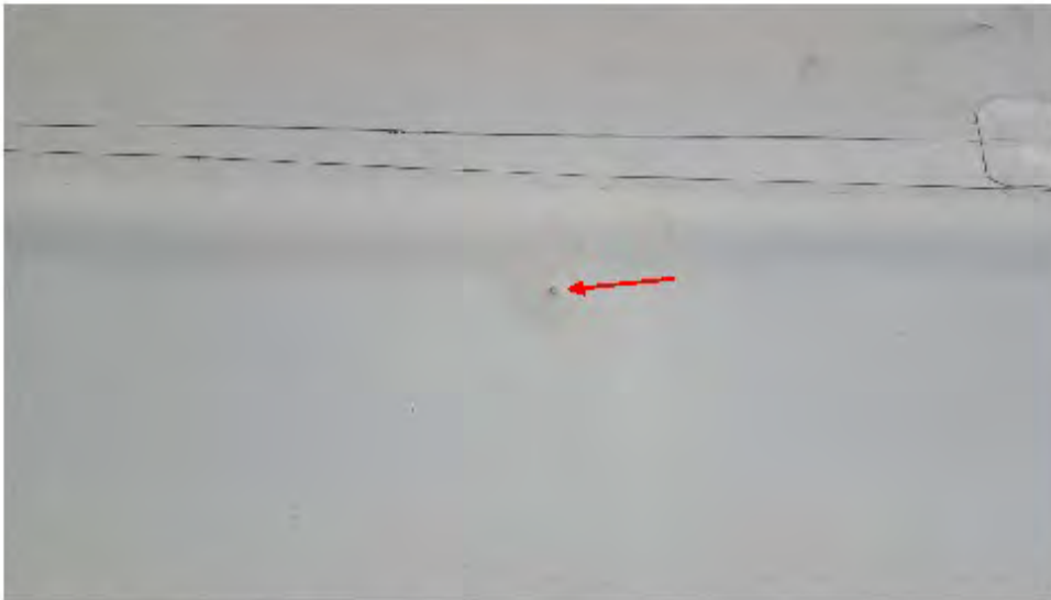
Backing out fasteners is damaging TPO
