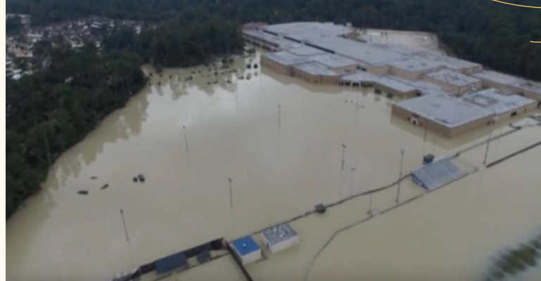
Harvey Flooding at Kingwood High School
