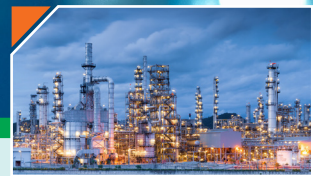
Hazardous Location Lighting
