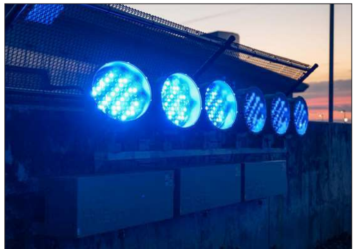
6 of the 24 color-changing luminaires lighting the Jefferson Street Viaduct.
