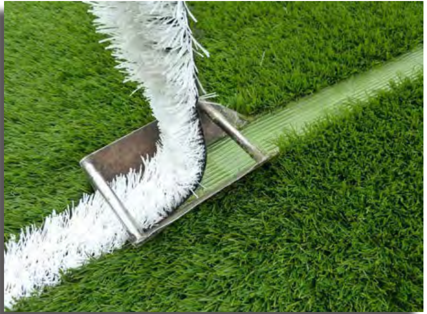
[ Figure 10: Inlay Installation ]
