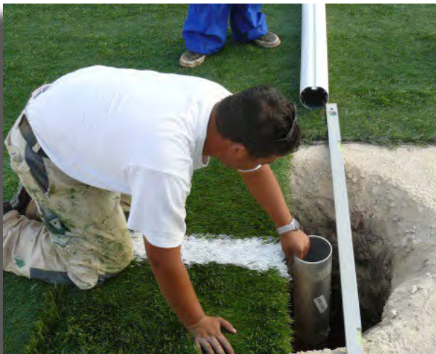
[ Fig. 12: Post Hole Positioning ]
